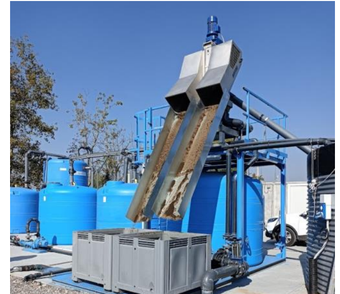
The slurry is first treated to remove coarse solids with a screw-press separator
