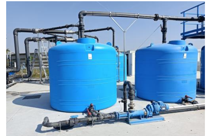
The slurry after the separation of the solids is placed in containers that feed the reactors where the process takes place
