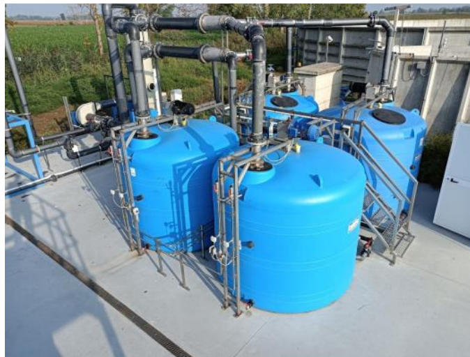
The scrubber cleans the ammonia-charged air exiting the reactors to form ammonium sulphate which can be used as a fertilizer
